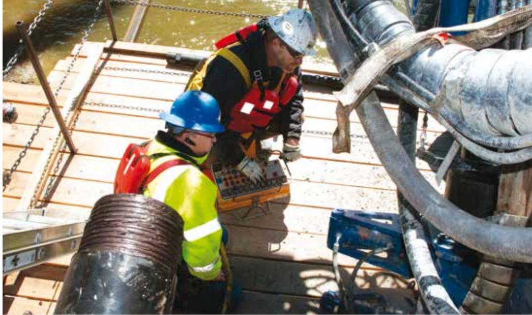
*(above) Stacy Lynn, of the Atlas Copco–Nashville store, is on site as GeoFirma owner and driller Eric Snyder begins the first of three 105-foot anchors. The anchors consist of stranded cable grouted into a 20-foot rock socket in the Cumberland River Park Stabilization Project at the park’s scenic overlook.*
