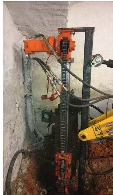
Pic.2: Drill works in progress with a lightweight mast at a room height of 1.50 m
