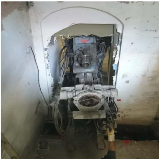
Pic. 1: Use of drill rig type "Hütte 202" in confined conditions
